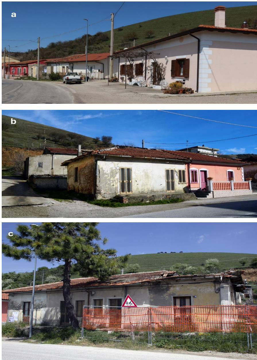
Figure 13: Bisaccia (Avellino province): the new constructions after the 1930 earthquake called “ Casette Asismiche- Aseismic Small Houses”. The Aseismic Houses show in figs a, b, c D date back to the 1930 post-earthquake fascist period and are still inhabited today (Photo by Spiga and Porfido [35, 55]).
