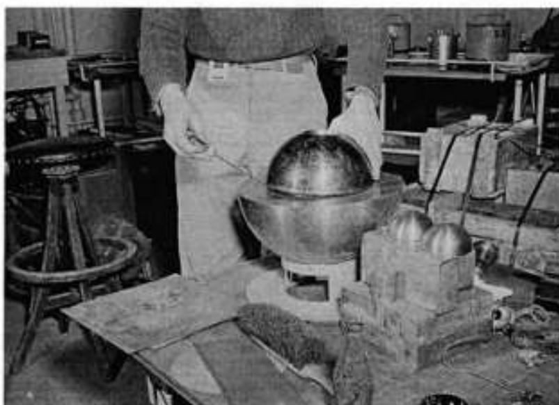
Slotin accident reconstruction assembly showing beryllium hemispheres. Note use of the screwdriver to hold the beryllium hemispheres apart and the two Pu hemispheres sitting atop the lead blocks. (LANL)
