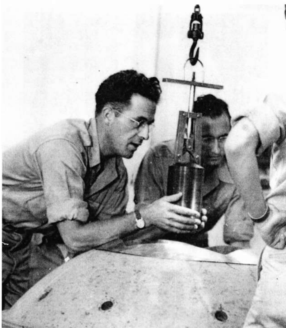
This very rare photo shows Raemer Schreiber steadying the 5" diameter Pu-filled uranium "capsule" as it is about to be loaded into the F-31 Fat Man Dural sphere inside Tinian Assembly Bldg. #3 in 1945. The top plate on this F-31 sphere is the same style as the one used on the Trinity sphere shown on the previous page. This top had a metal funnel built into it to protect the surrounding explosive blocks while it was being loaded into the 8.75" diameter Uranium tamper sphere down in the very center of that sphere. Schreiber was present a few weeks earlier in the McDonald Ranch House to observe the assembly of that same style capsule for the Trinity device. In an extensive 1996 interview, he gave the author a complete description of exactly how that capsule was assembled. (Author)
