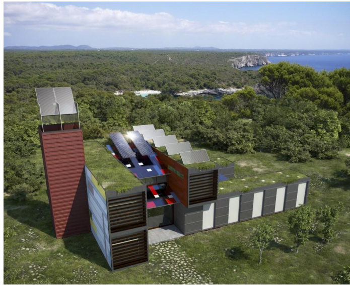
Figure 2: R4House has been built using Six Modules, and all its Components are Removable, Including Foundations, Installations and Equipment
