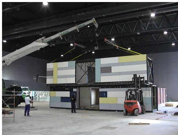
Figure 7: The 6 Partially Manufactured Modules were ensembled in just one day
