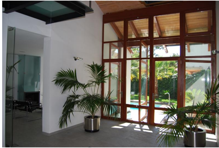
Figure 11: Interior of Torres house. The Covered Central Courtyard can be seen, Which Cools all Rooms in Summer and Warms them in Winter. The Double-Glazed Entrance is also Noticeable. In Summer, there is Only One Glass door, and in Winter, There are Two Glass Doors Forming a Greenhouse at the Entrance to the House.
