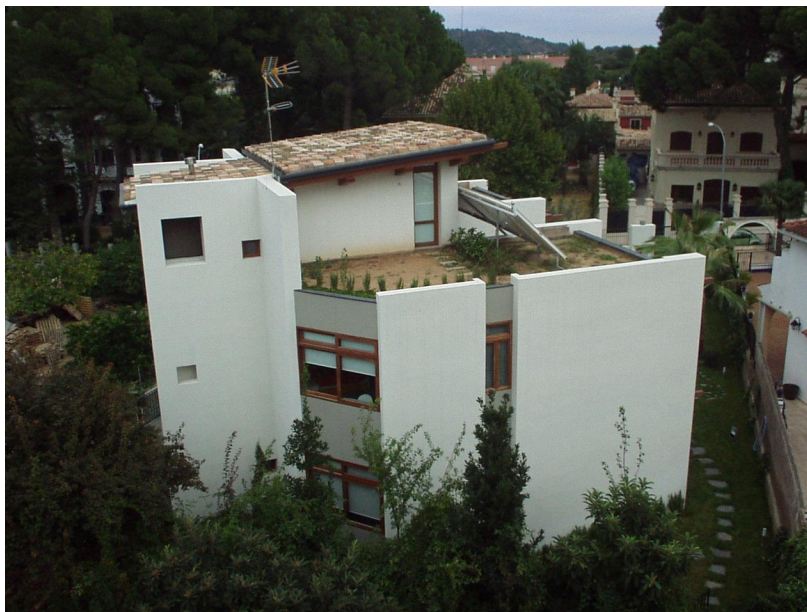
Figure 4: The Torres House's Garden Roof. On the North Side, the Wind Catcher can be seen, which Collects Cool Air Coming from the East, Transports it to a Series of Underground Galleries Located below the Basement, where its Temperature is Lowered before it Enters the House to Cool it in the Summer
